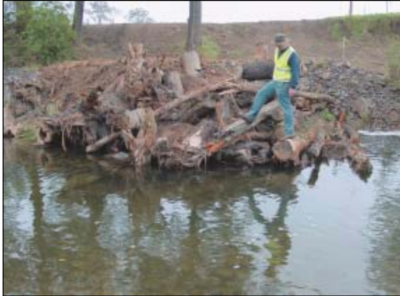
Figure 24. Deflector jam installed on the Williams River, NSW, Australia. From Brooks et al. (2006).
