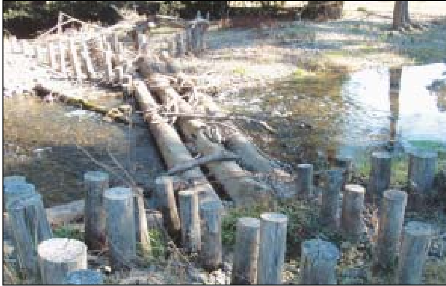
Figure 27. Log sill bed-control structure installed on the Orara River, NSW, Australia. From Brooks et al. (2006).
