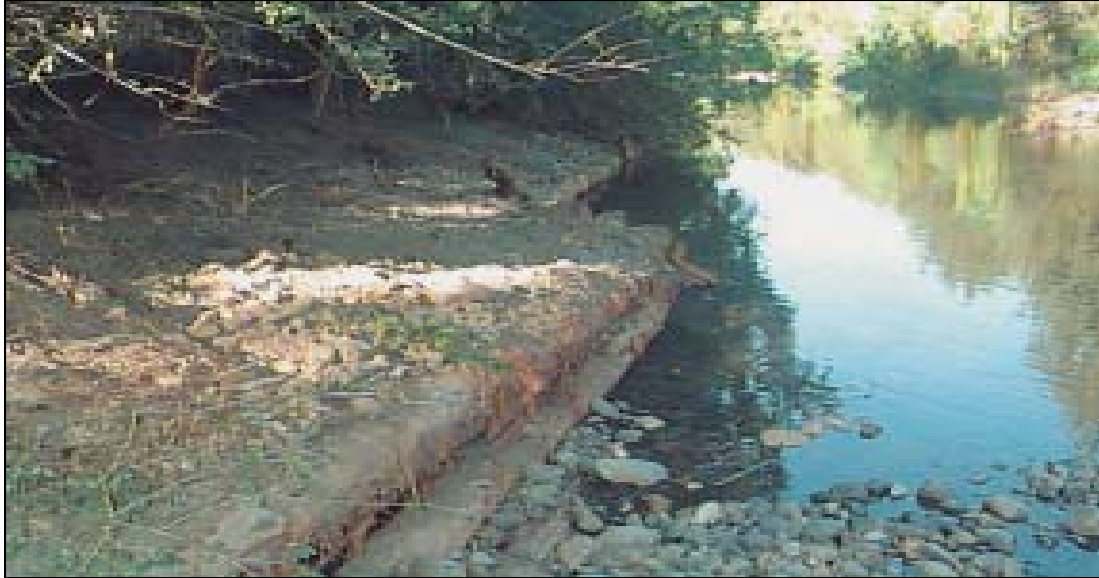
Figure 26. Bank revetment structure installed on the Williams River, NSW, Australia. From Brooks et al. (2006).
