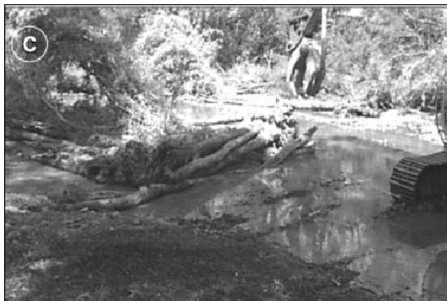
Figure 25. Bar apex jam installed on the Williams River, NSW, Australia. From Brooks et al. (2006).
