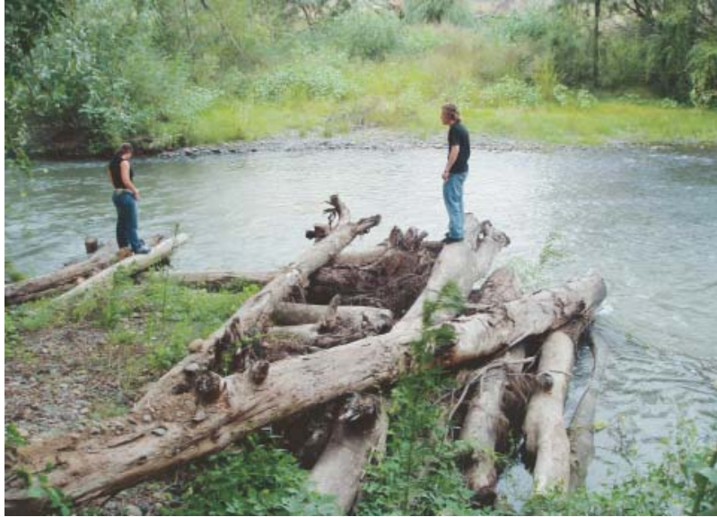
Figure 22. An ELJ designed to provide bank stability. From Brooks et al. (2006).
